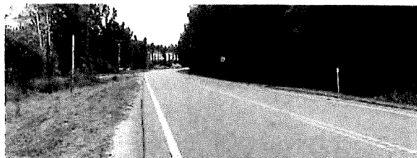
Substandard shoulder at CR 108 near Pineridge Drive
